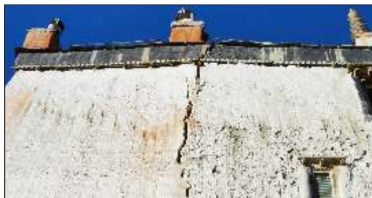
Cracked wall of Lo Manthang Palace. Photo: Ghanshyam Khadka/NIMJN
